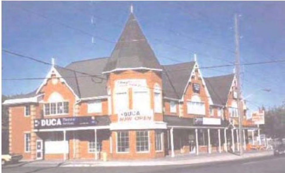
Figure X4.19: Taller structure anchoring street corner
