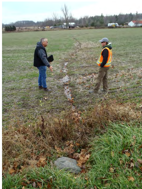
Photo 23. Upstream extent, looking downstream.
