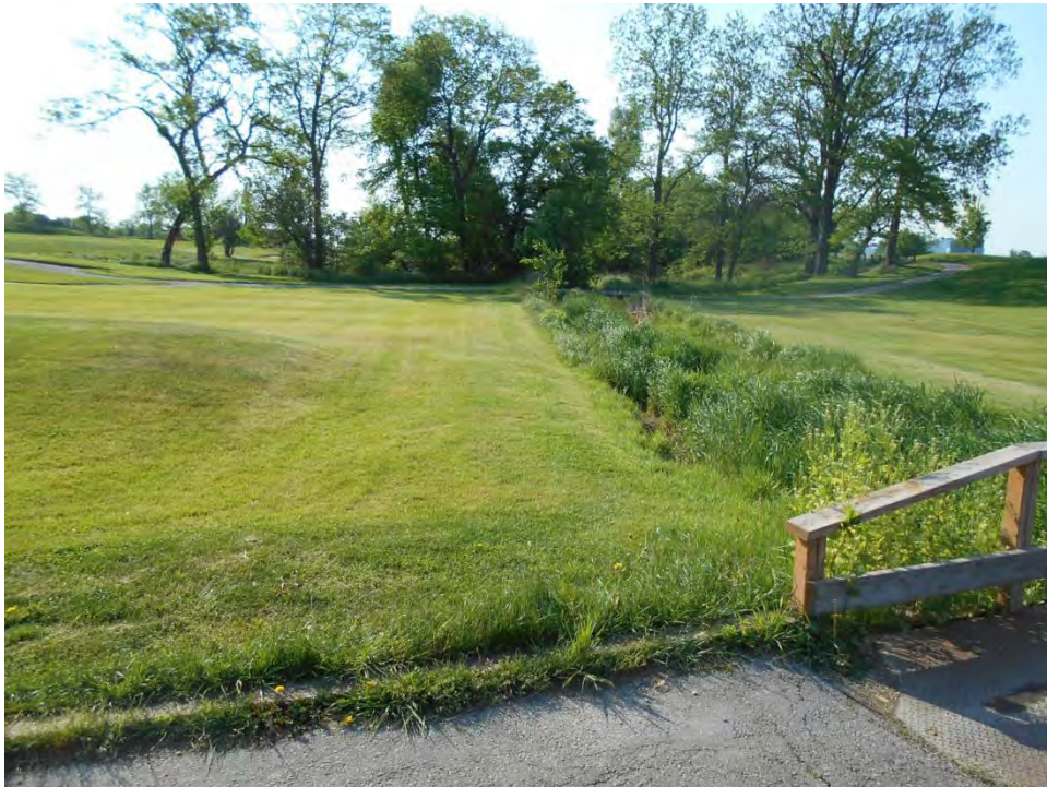
Photo 8. Cart path (on the downstream end), looking downstream.
