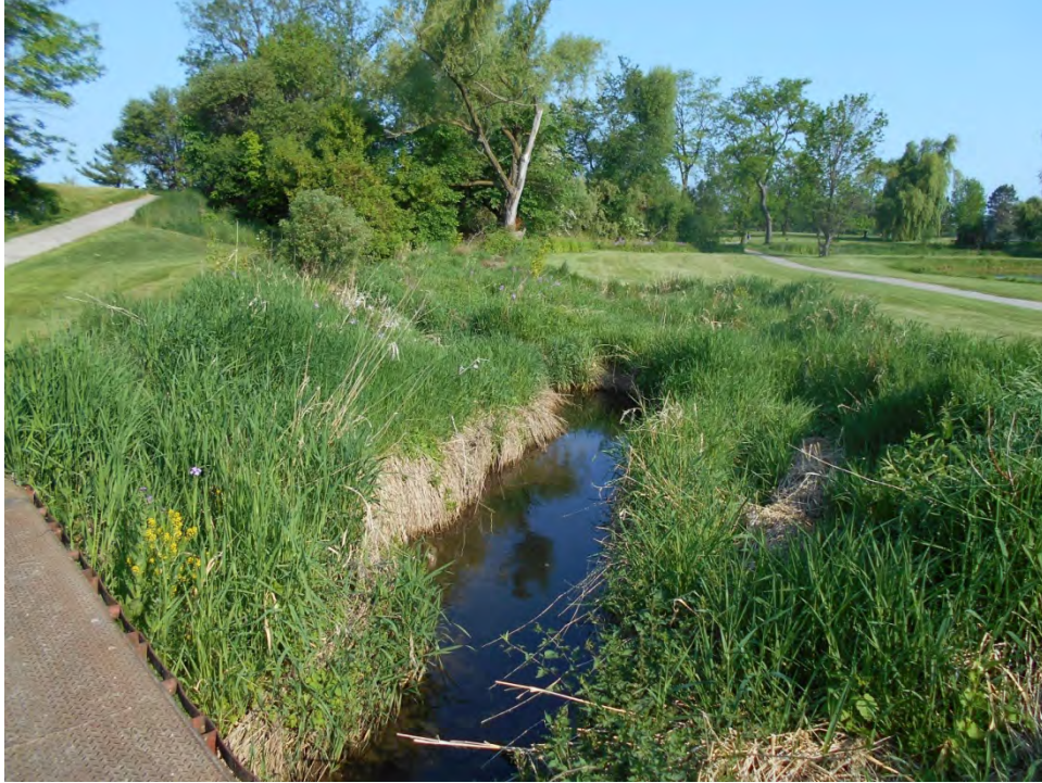
Photo 12. Downstream extent (cart path), looking upstream.
