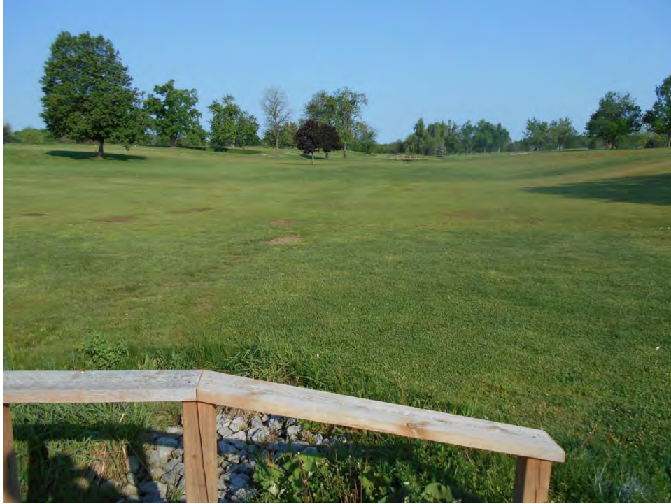
Photo 7. Cart path (on the downstream end), looking upstream.
