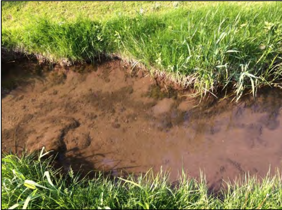
52. E-T1-3 Silt accumulation in multiple areas of the channel.
