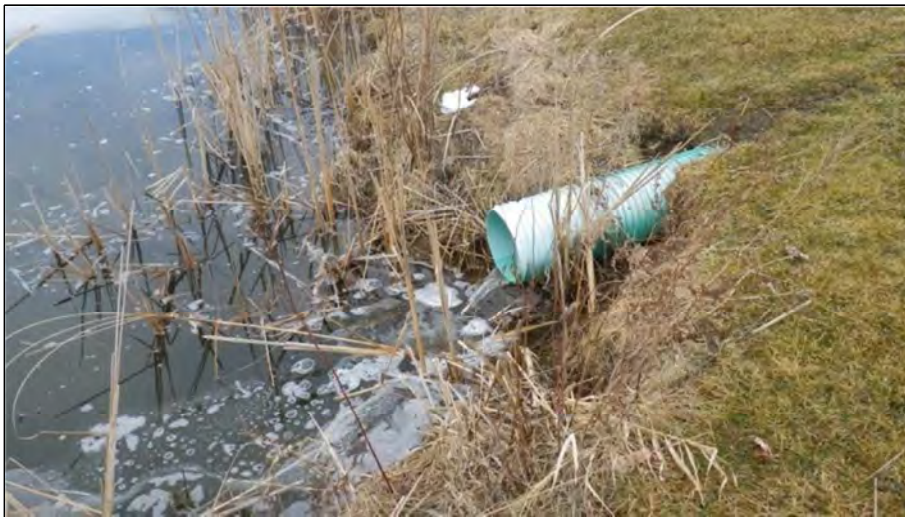
98. HDF -4. Outlet at golf course pond downstream end. Feature type is swale and flow condition is surface flow minimal.
