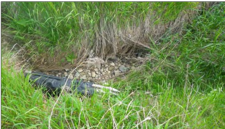
58. HT -2b -4 (Segment 2) . Downstream of confluence with roadside ditch, features combine to establish defined bed and banks approaching culvert.
