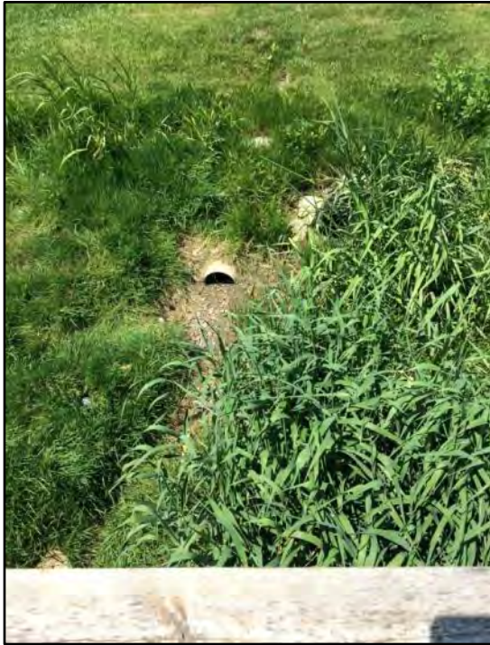
44. E-T1-4 Channel alternates between being piped under golf course fairways (as seen in this photograph) and being a grassed trapezoidal channel.
