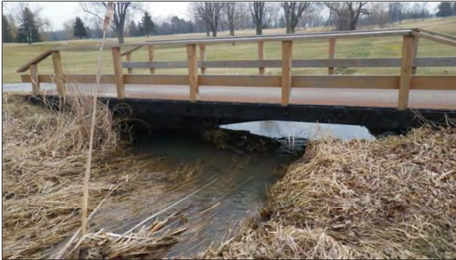
67. E -T1 -4 (Segment 1). At first cart path crossing, facing downstream. Water flows beneath bridge and drains into small pipe across the fairway. Feature type is classified as tiled drainage (buried stream/pipe) because the feature is primarily piped through the extent of the golf course. Flow condition is surface flow substantial.
