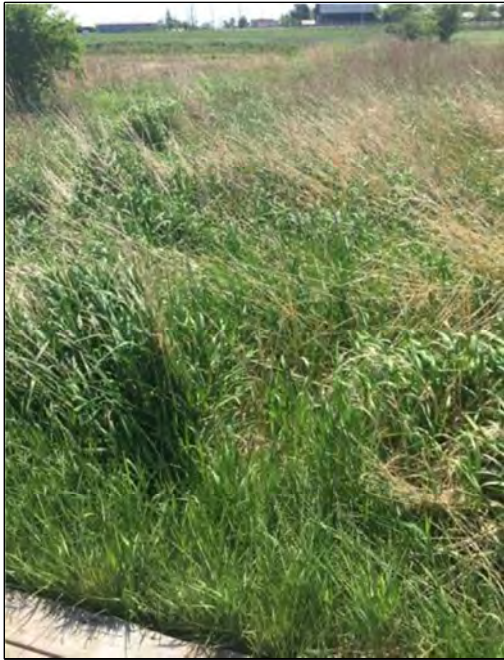
29. HT -2b -2 (Segment 2). Upstream end of Segment located at small boardwalk. Visible depression through this Segment. Feature type is swale and flow condition is no surface water.
