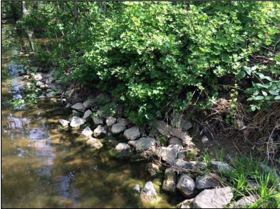
82. HT-2a-2 Rip rap placed along toe of right bank protecting private property.
