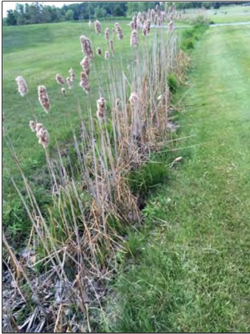
111. HDF -3. Facing upstream, near downstream end of feature. Feature heavily vegetated with cattails. Feature type is swale; flow condition is no surface water.
