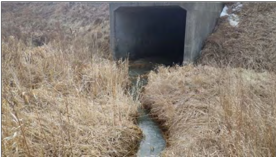
34. HT -2b -2 (Segment 3). Facing downstream to culvert at Trafalgar Road, note well -defined channel banks. Feature type is defined natural channel (visible banks); flow condition is surface flow substantial.
