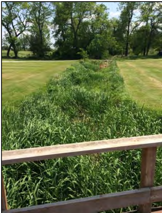
45. E-T1-4 Channel alternates between being piped under golf course fairways and being an intermittent grassed trapezoidal channel (as seen in this photograph).
