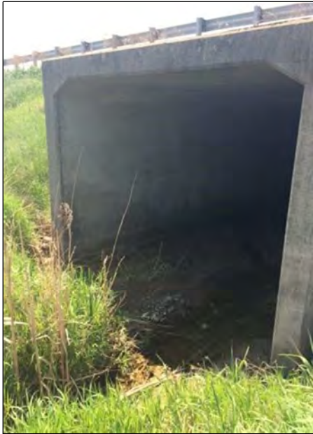
41. HT -2b -2 (Segment 3). Standing water in culvert, downstream end of Segment. Feature type is defined natural channel (visible banks); flow condition is no surface. Management Recommendation: None. Feature is classified as a Watercourse
