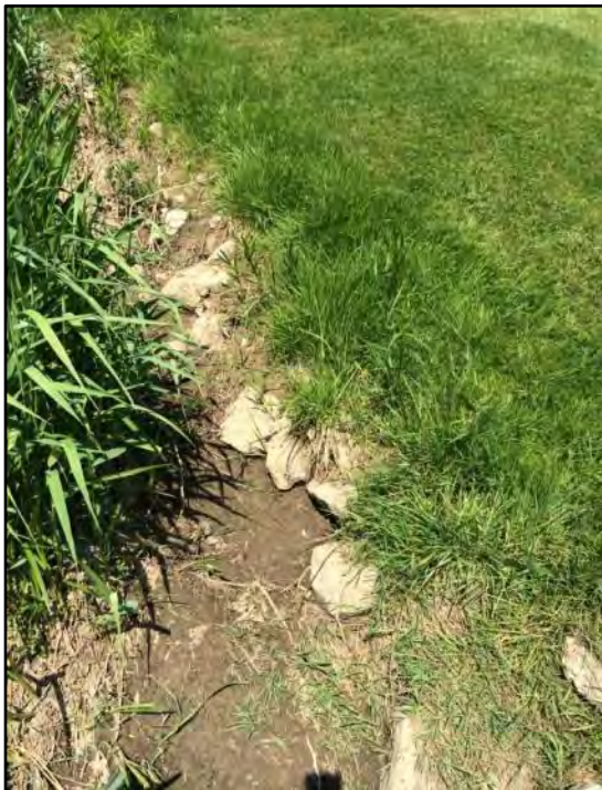
43. E-T1-4 Channel is dry and armouring placed along left bank placed to prevent erosion along fairway boundary.
