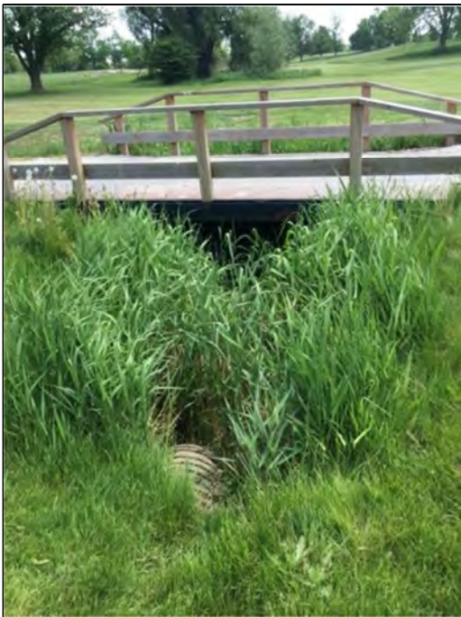
78. E -T1 -4 (Segment 1). Pipe outlet at second cart path crossing, facing downstream. No water noted. Feature type is classified as tiled drainage; flow condition is no surface water.
