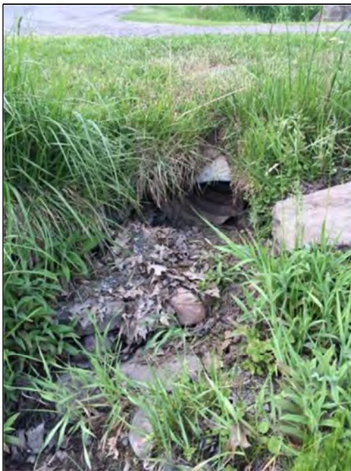
137. W -T1 -2b (Segment 1). Upstream end of feature, some erosion due to CSP outlet. Feature type is swale and flow condition is no surface water.
