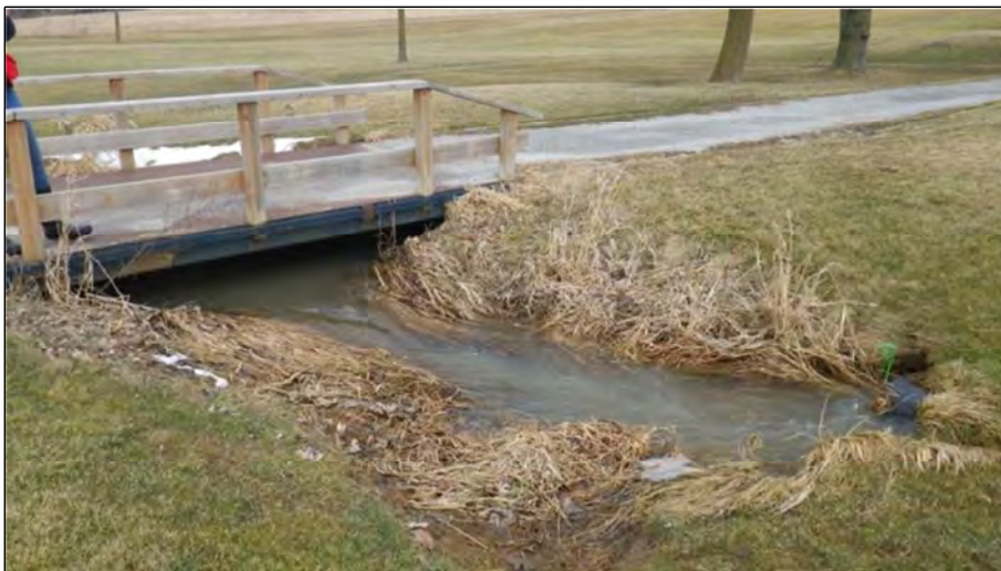
68. E -T1 -4 (Segment 1). Downstream side of second cart path crossing. Water flows out of pipe upstream of cart path crossing and then again drains into pipe to traverse another fairway. Feature type is classified as tiled drainage (buried stream/pipe) because the feature is primarily piped through the extent of the golf course. Flow condition is surface flow substantial.
