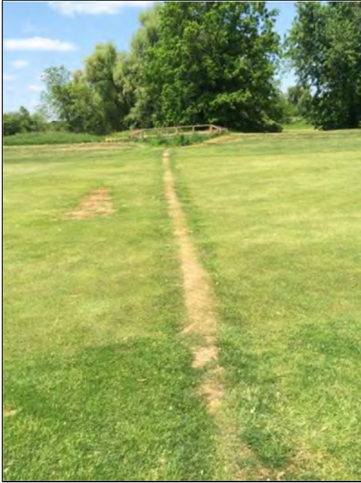
77. E -T1 -4 (Segment 1). Facing upstream towards first cart path crossing, feature is piped, no surface flow. Feature type is classified as tiled drainage; flow condition is no surface water.
