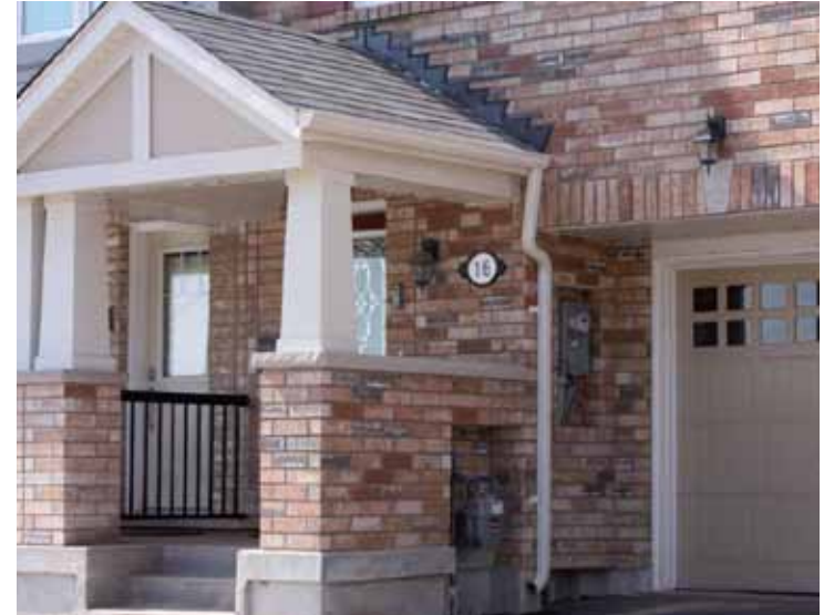
SCREENED UTILITY METERS
