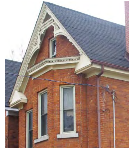
Window lintels and sills, window shutters, wood and stone detailing and facades with vertically oriented windows are important character components of residential buildings in the Hamlet.
