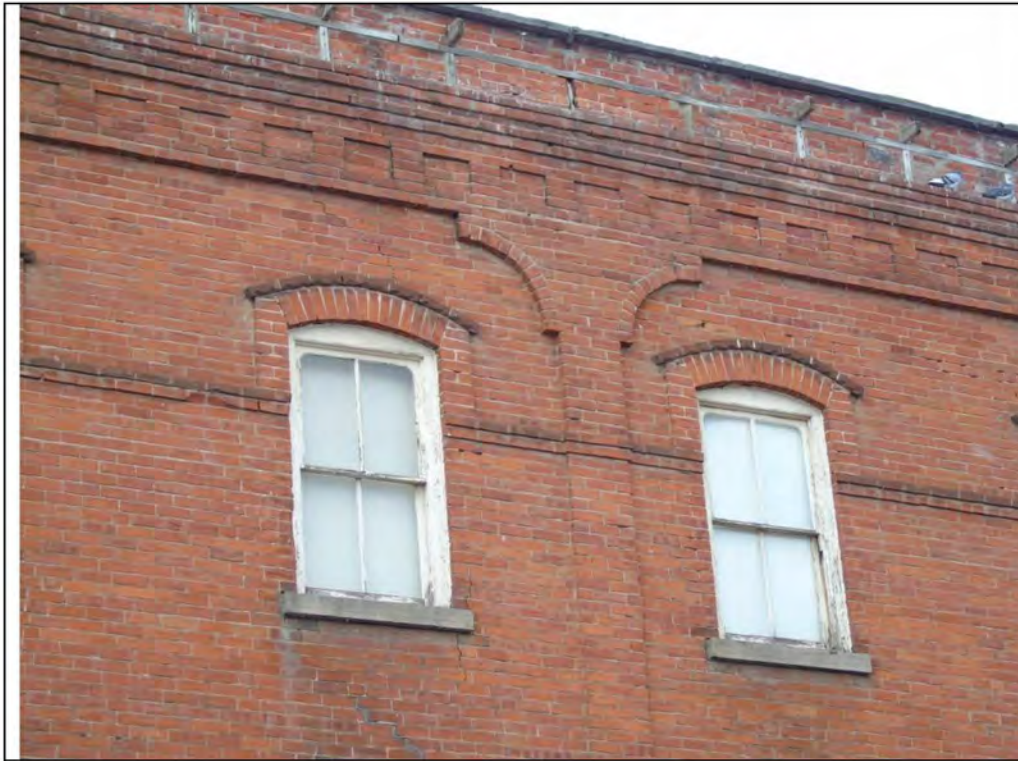
Plate 49: South elevation of 79 Main Street South, showing decorative brickwork, sash windows with segmental arches, and repairs to the roofline, looking northeast.
