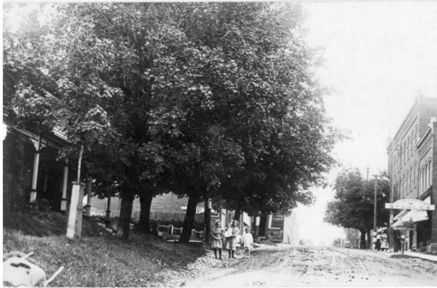
Figure 11: View up the Mill Street hill towards Main Street, circa 1908 (Esquesing Historical Society #21522).
