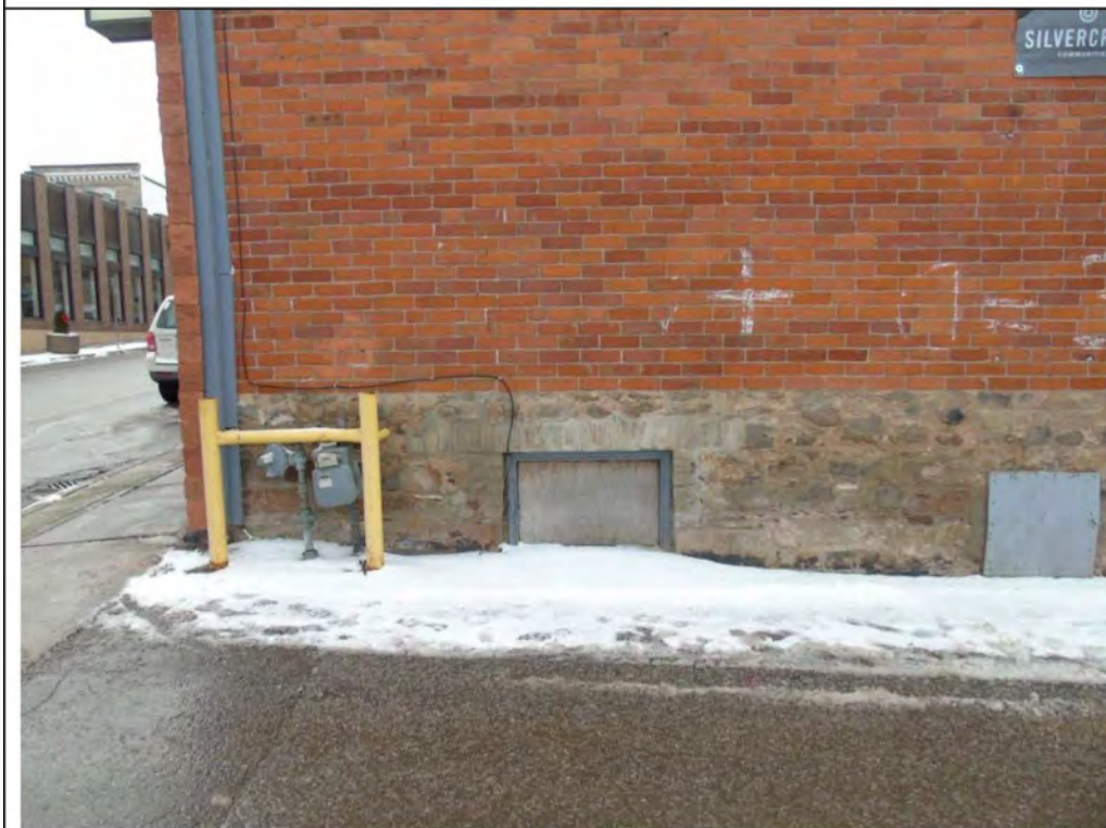
Plate 22: Detail of the brickwork and foundation on the east elevation of the structure at 94-96 Mill Street, looking west.
