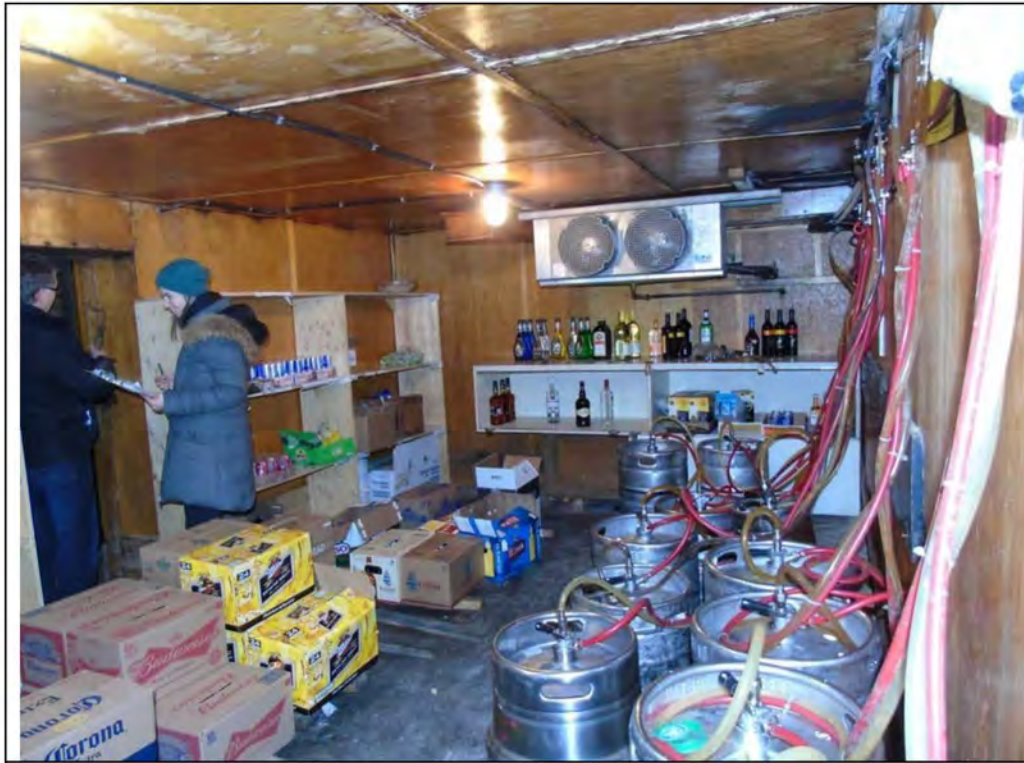
Plate 67: Basement of 71- 77 and 79 Main Street South, showing modern refrigeration facilities for the restaurant and bar.
