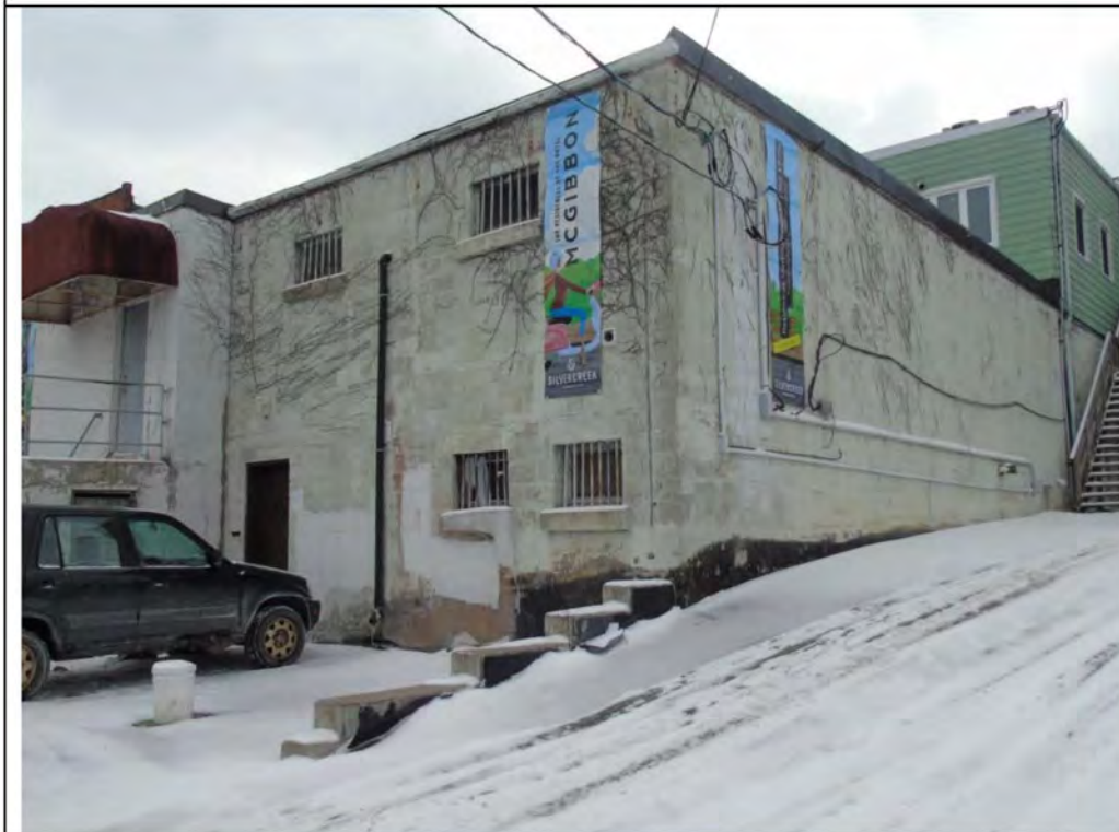
Plate 6: East and north elevations of the concrete block addition at 69 Main Street South, looking southwest.
