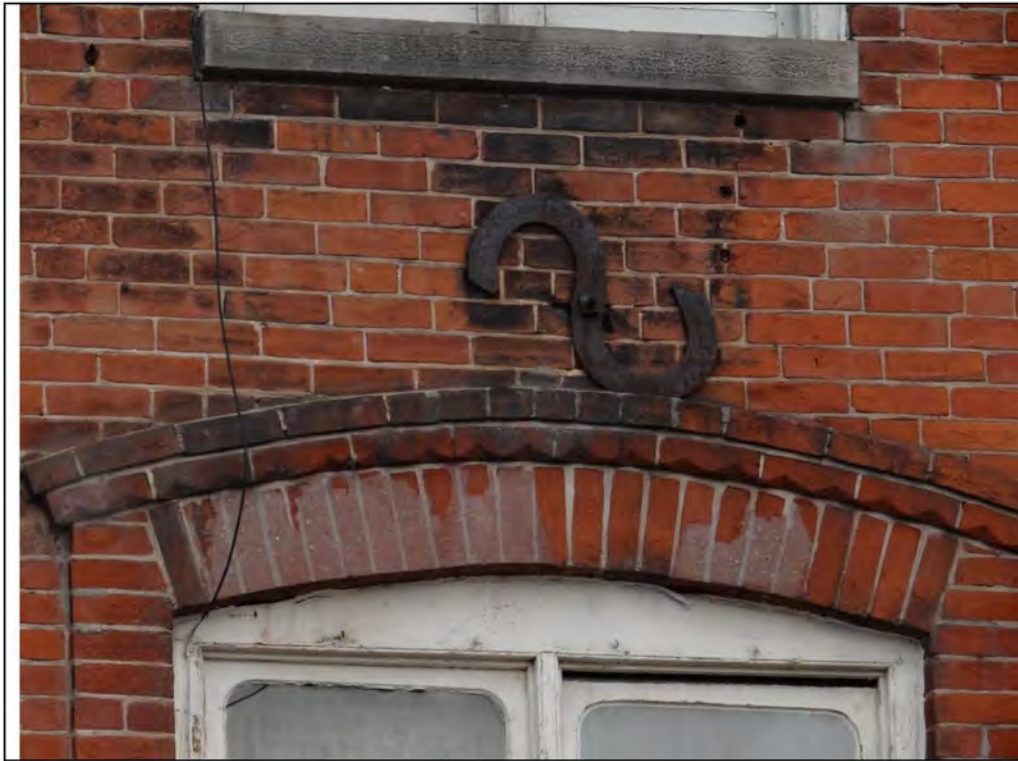
Plate 45: West elevation of 79 Main Street South, showing segmental arches on the window and decorative metal tie-ends, looking east.
