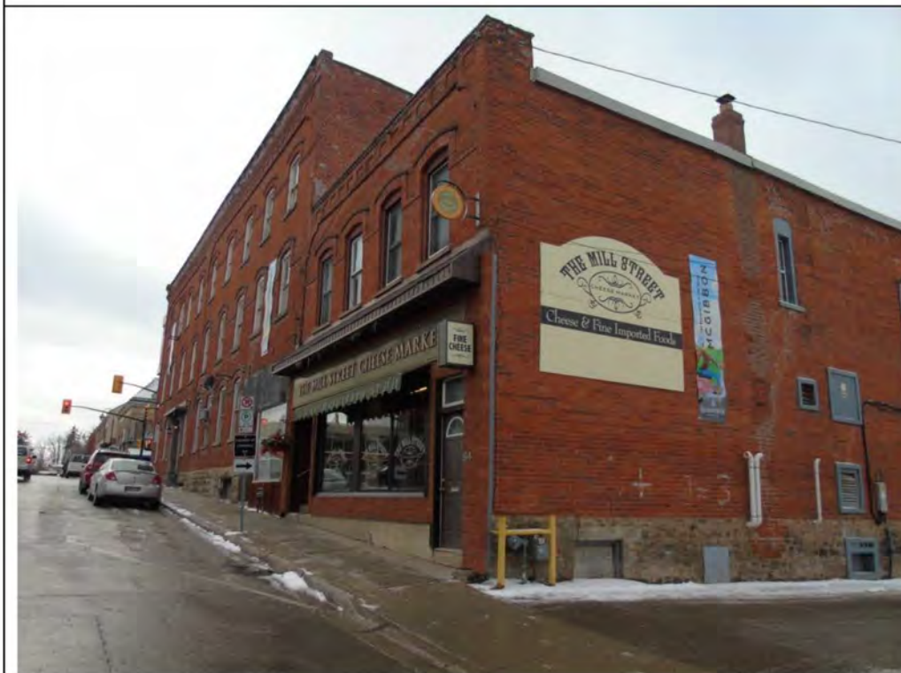
Plate 20: South and east elevations of the structure at 94-96 Mill Street, looking northwest.
