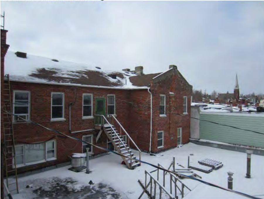
Photo #6: Side of the building
