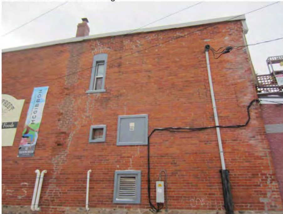
Photo #4: Back of the building
