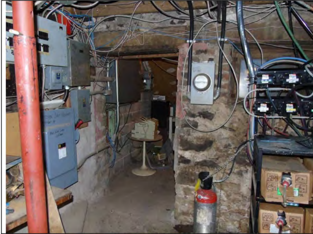
Plate 65: Basement of 79 Main Street South, showing stone foundations, hewn beams, and modern electrical panels.
