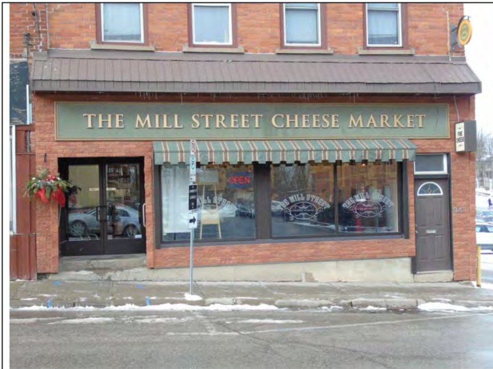
Plate 19: Detail of the brick work and large windows on the first floor of the south elevation of the structure at 94-96 Mill Street, looking north.
