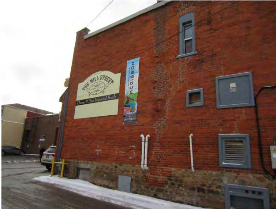
Photo #3: Back of the building
