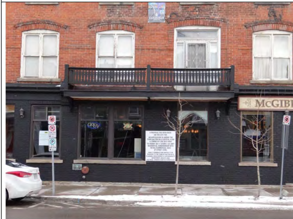
Plate 46: West elevation of 79 Main Street South, showing ground level windows and brickwork, looking east.
