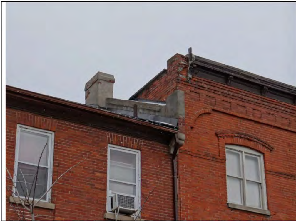
Plate 33: West elevation of 71-77 Main Street South showing stepped parapet separating the structure from attached 79 Main Street South, looking northeast.
