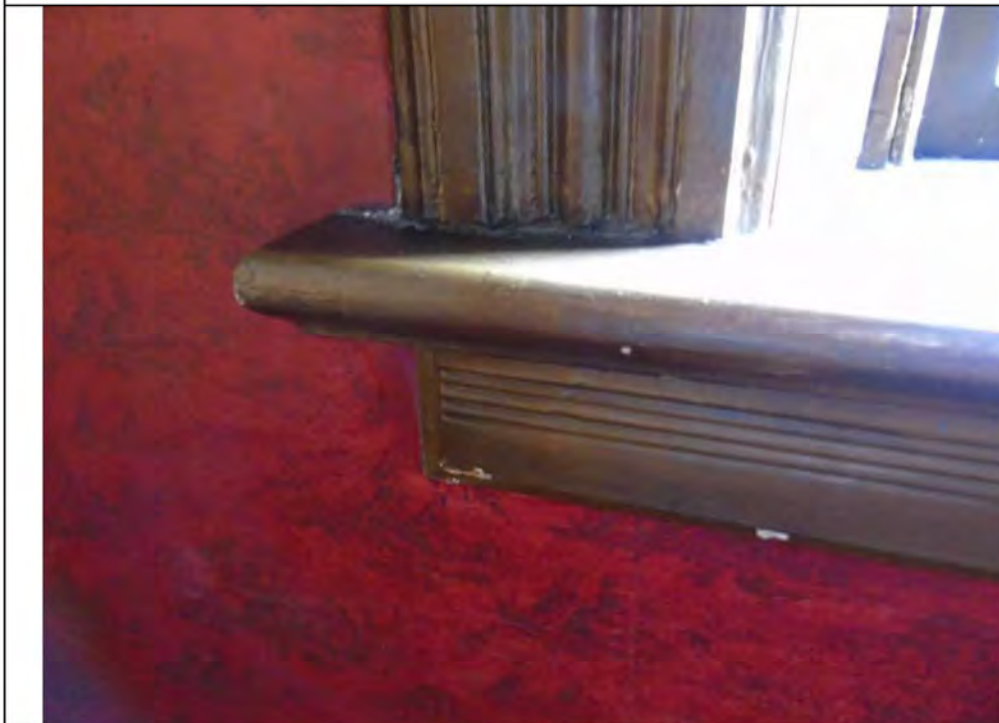
Plate 54: Detail of window sill and trim in the restaurant.
