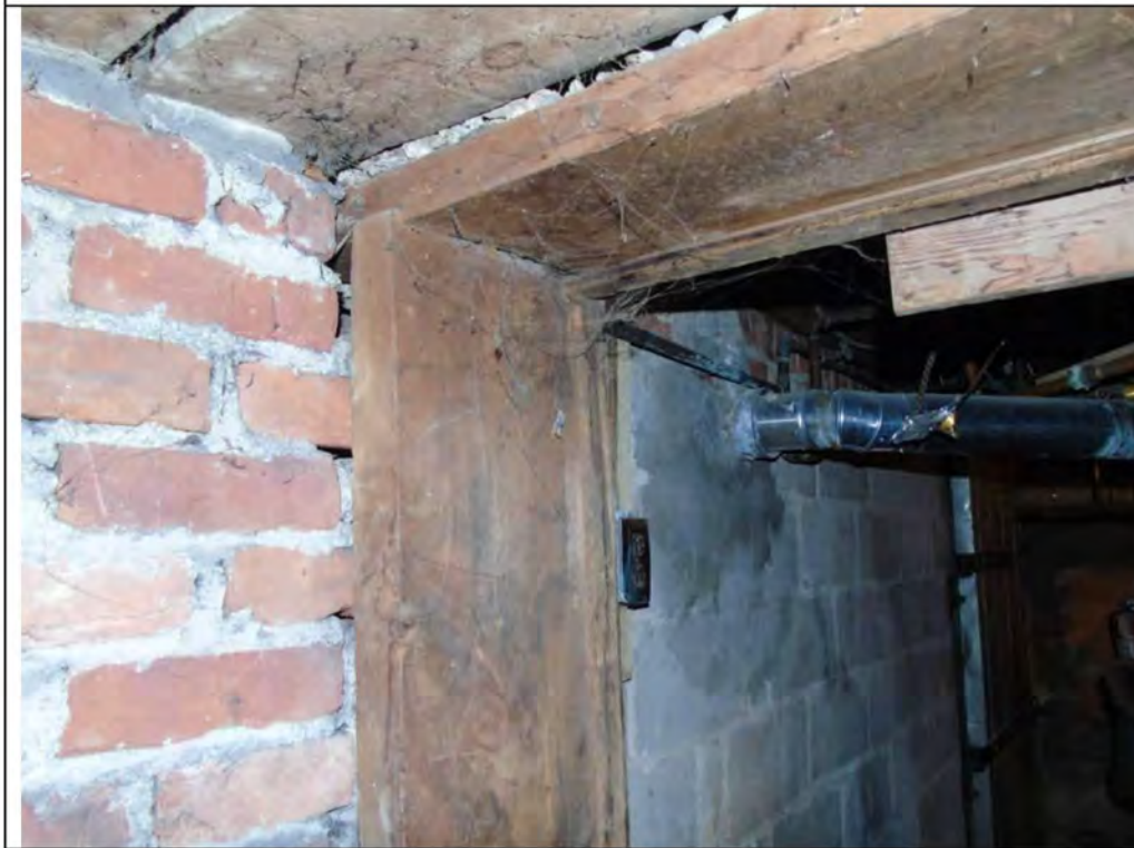
Plate 70: Basement of 71- 77 and 79 Main Street South, showing red brick and cinder block foundations, softwood floorboards, and modern dimensional lumber door framing.
