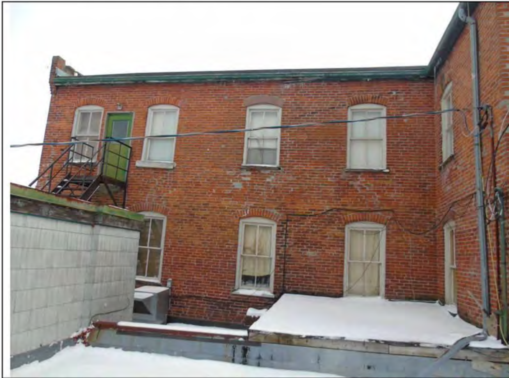
Plate 51: South elevation of 79 Main Street South, showing the eastern ground level retail space, looking north.
