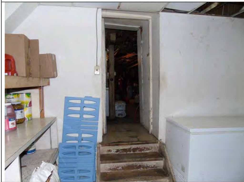
Plate 68: Basement of 71- 77 and 79 Main Street South, showing modern drywall and ceiling tiles in a food storage area.
