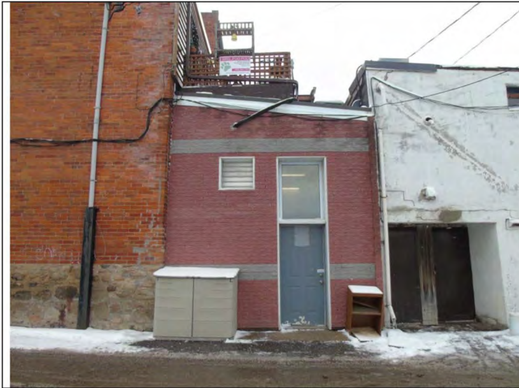
Plate 23: Detail of the east elevation of the northern addition and second floor patio at 94-96 Mill Street, looking west
