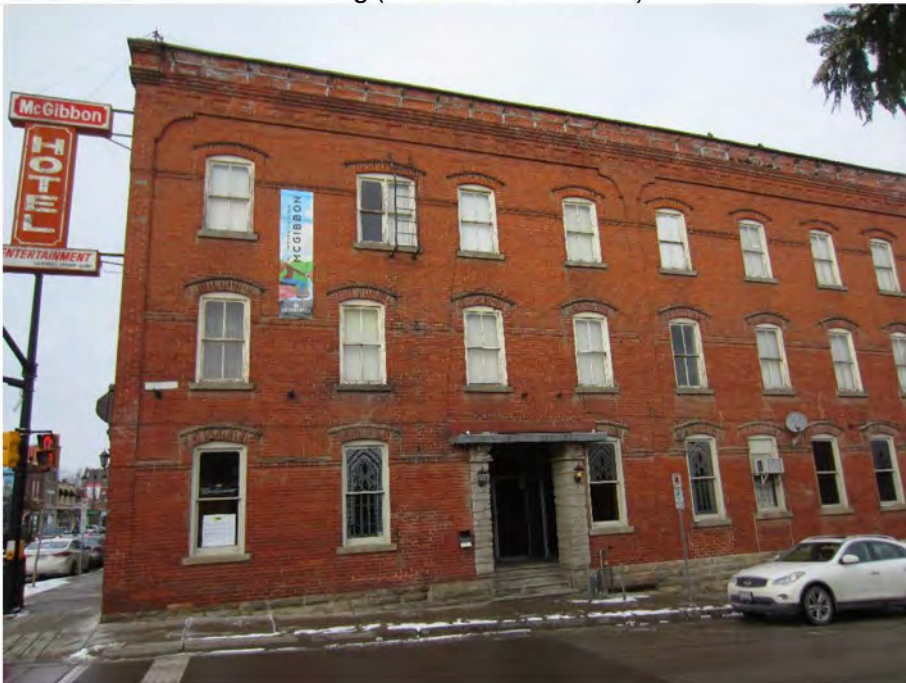
Photo #2: Side of the building (on Mill Street)
