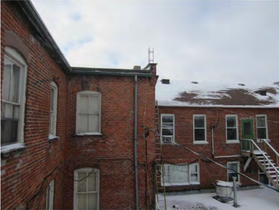
Photo #5: Side of the building
