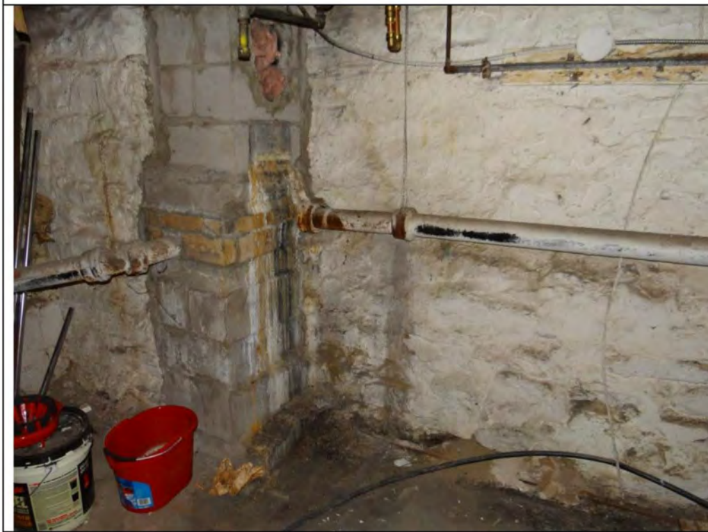
Plate 12: Detail of the stone foundations in the basement of 69 Main Street South.
