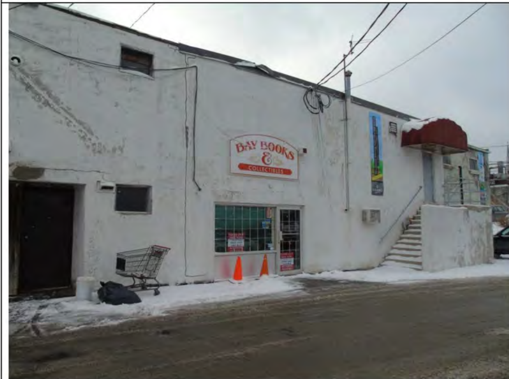
Plate 36: East elevation of the eastern addition of 71-77 Main Street South fronting on parking lot, looking northwest.
