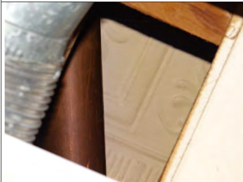
Plate 8: Detail of stamped tin ceiling tiles on original main floor ceiling of 69 Main Street South.
