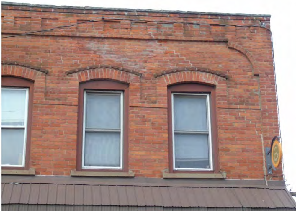
Plate 18: Details of the second floor fenestration and decorative brickwork on the south elevation of the structure at 94-96 Mill Street, looking north.
