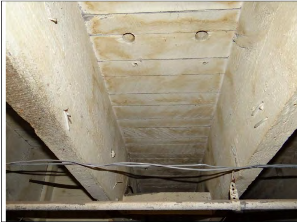
Plate 13: Detail of the sawn floor joists and softwood plank flooring from the basement of 69 Main Street South.
