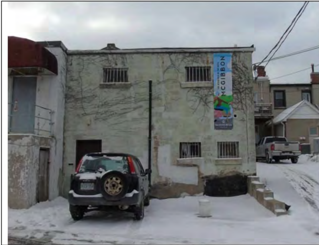
Plate 7: East elevation of the concrete block addition at 69 Main Street South, looking west.
