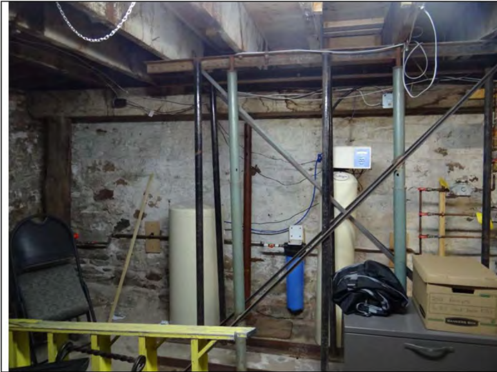
Plate 31: Detail of modern structural steel posts added to reinforce the main floor joists in the basement at 94-96 Mill Street.
