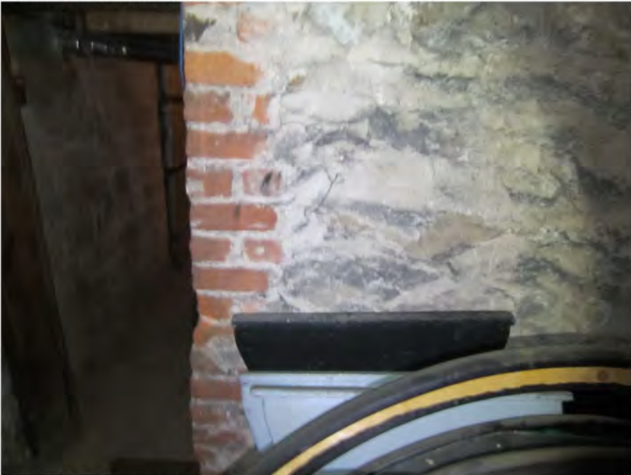
Photo #12: Basement brick foundation
