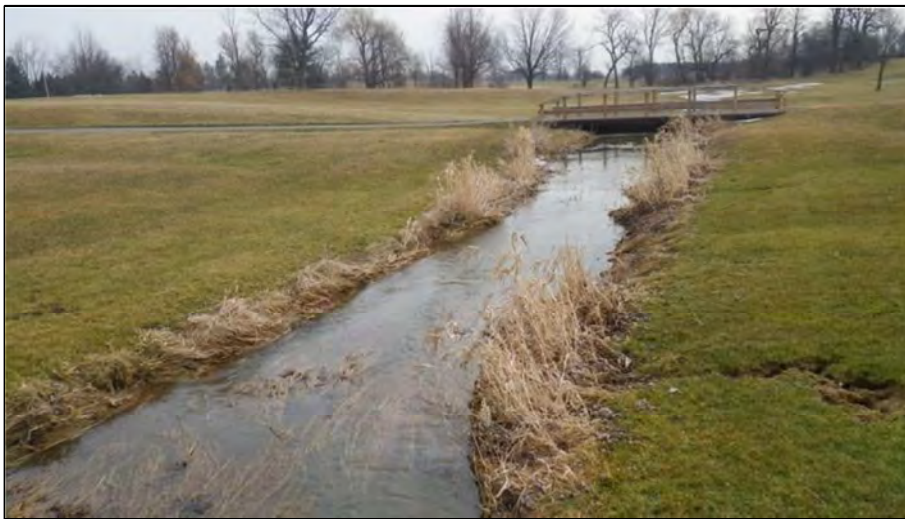
72. E -T1 -4 (Segment 1). Facing downstream towards fourth cart path crossing. Water flows at surface after outletting from pipe. Feature type is classified as tiled drainage (buried stream/pipe) because the feature is primarily piped through the extent of the golf course. Flow condition is surface flow substantial.
