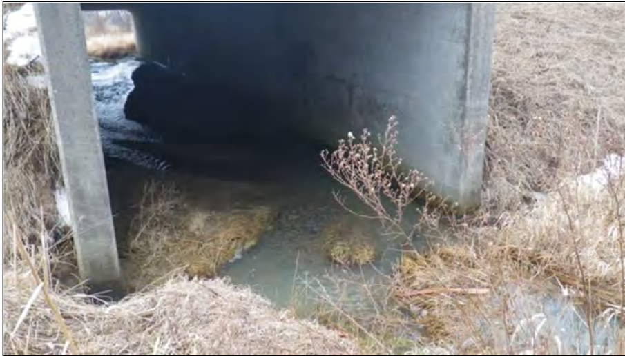
35. HT -2b -2 (Segment 3). Downstream end of Segment where feature enters Trafalgar Road culvert. Feature type is defined natural channel (visible banks); flow condition is surface flow substantial.
