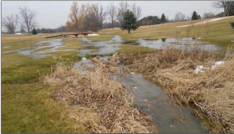
71. E -T1 -4 (Segment 1). Facing upstream towards third cart path crossing. In background of photo water is pooling at surface where it has overwhelmed the pipe. In foreground, pipe outlets into grasses area, where flow is relatively fast and erosion has occurred around the outlet. Wetted depth is 14cm. Feature type is classified as tiled drainage (buried stream/pipe) because the feature is primarily piped through the extent of the golf course. Flow condition is surface flow substantial.
