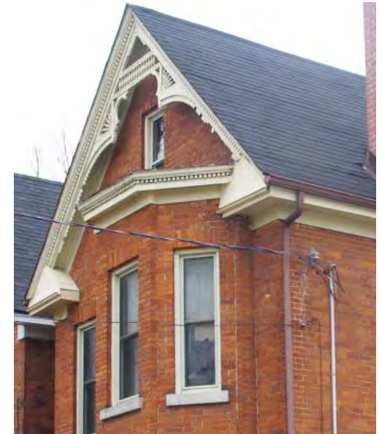
Window lintels and sills, window shutters, wood and stone detailing and facades with vertically oriented windows are important character components of residential buildings in the Hamlet.
