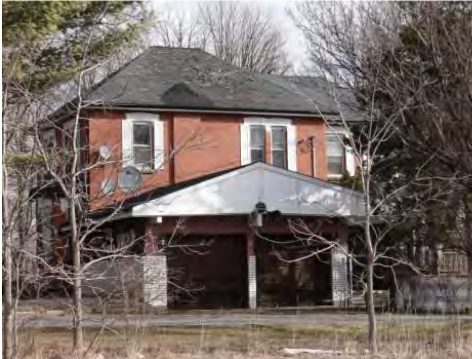
West elevation of the residence, looking east from shopping center parking lot.
