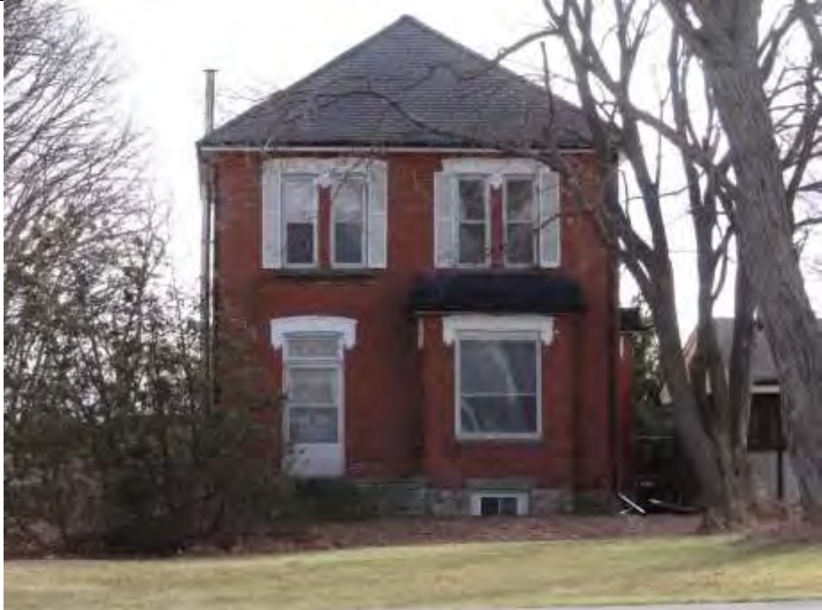
North elevation of the residence, looking south from Steeles Avenue.
