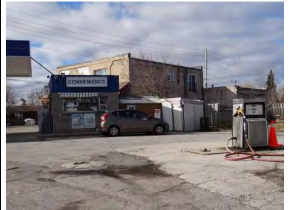
East elevation, looking northwest.
