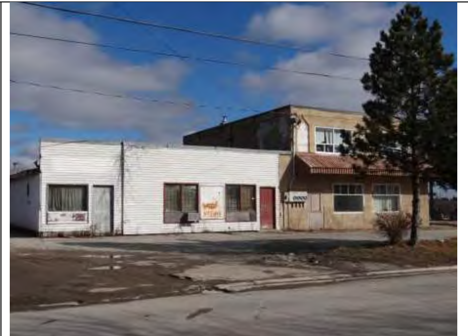
North and west elevation, looking east.
