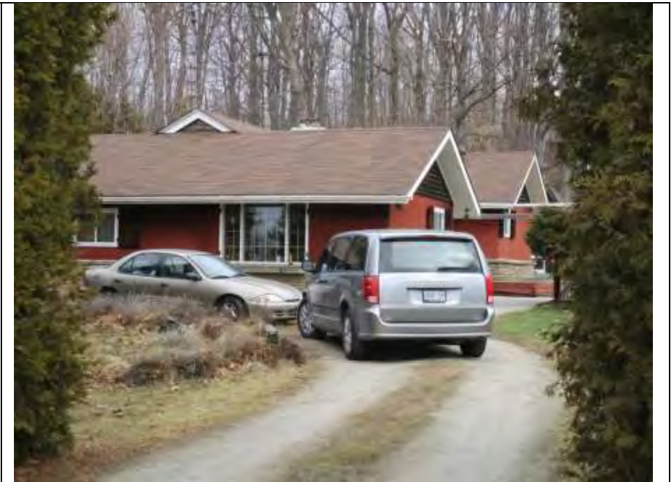
West and south elevations, looking east.
