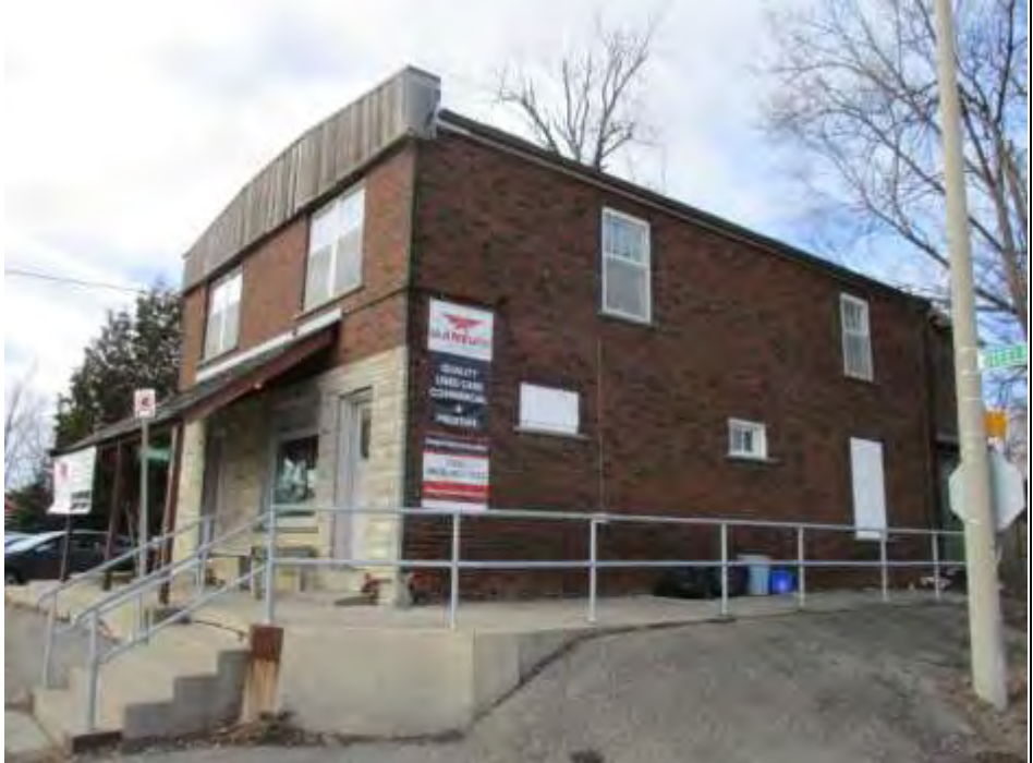
South and east elevation, looking northwest.
