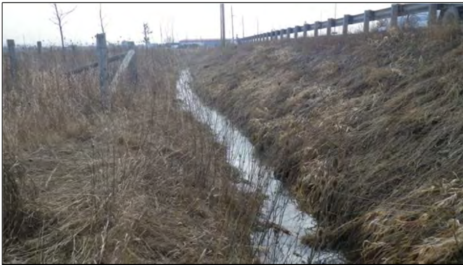
48. Roadside ditch along Trafalgar adjacent HT -2b -4 (Segment 1). Standing water.
