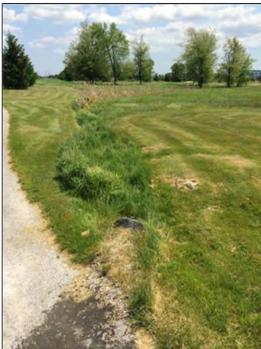
100. HDF -4. Facing upstream, area where feature is densely vegetated with cattails and grasses before entering a pipe. Feature type is swale and flow condition is no surface water.
