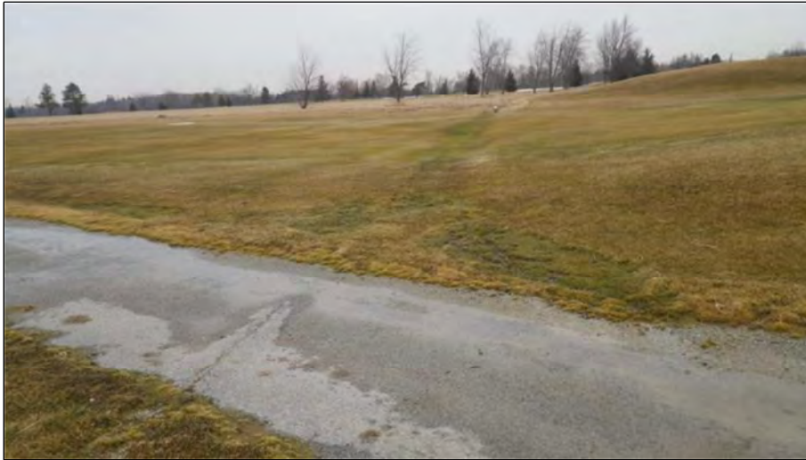
97. HDF -4. Facing upstream from downstream end of feature. Feature is piped to the downstream outlet at a pond. Feature type is swale and flow condition is surface flow minimal.
