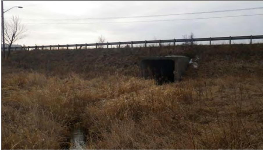
33. HT -2b -2 (Segment 3). Facing downstream to culvert at Trafalgar Road, note overhanging grasses. Feature type is defined natural channel (visible banks); flow condition is surface flow substantial.
