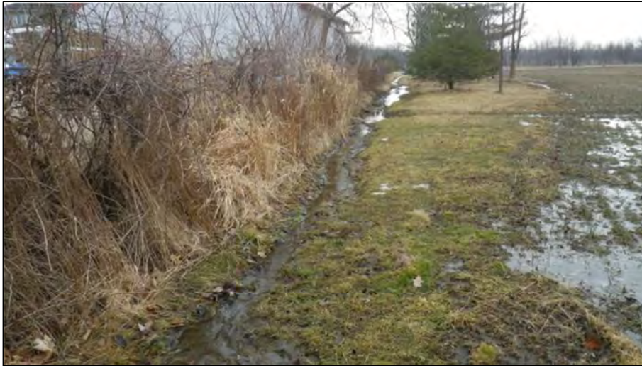
136. W -T1 -2b (Segment 1). Downstream end of feature. Feature makes a turn westward and drains towards Sixth line. Feature type is swale and flow condition is surface flow minimal.
