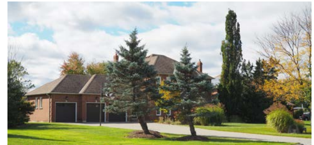
③ Dwelling on Oak Ridge Drive, adjacent to the subject site.
