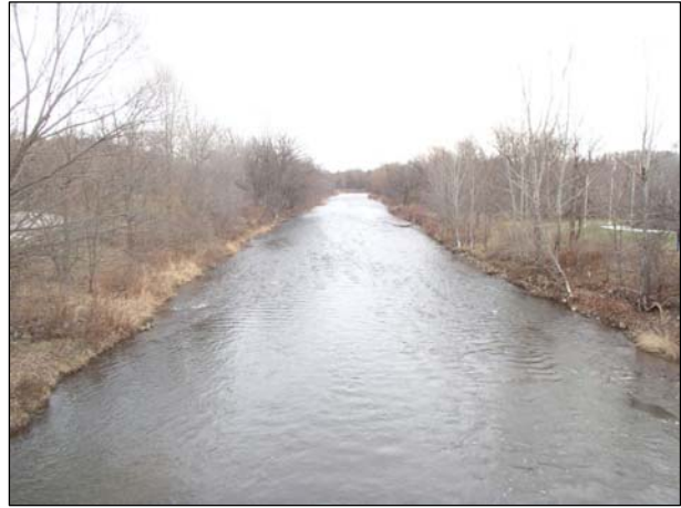
Photo 2: Main Street bridge looking downstream
