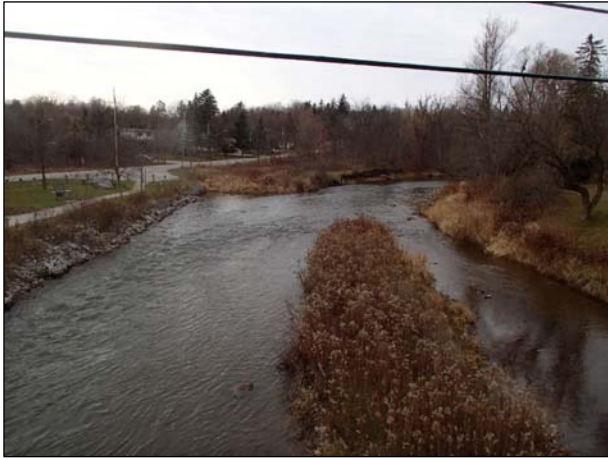
Photo 1: Main Street bridge looking upstream
