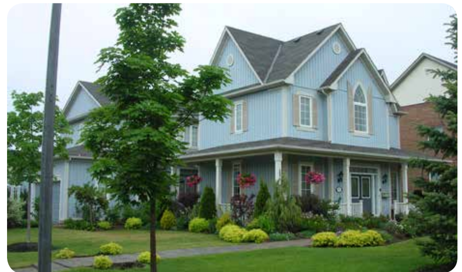
Corner lot houses should have architectural features that address both street frontages.
