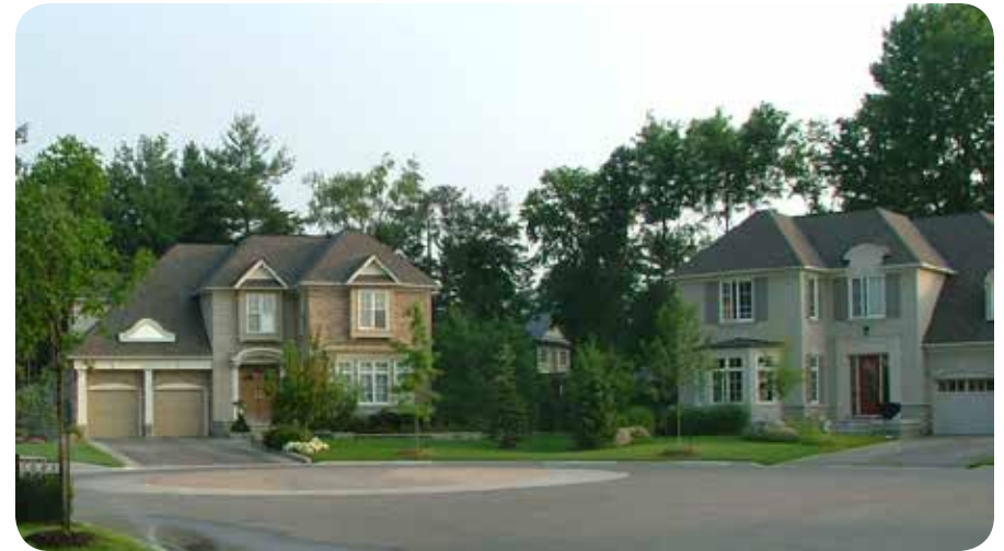
On elbow lots, locate driveways away from the centre viewpoint to create visually attractive streetscapes.
