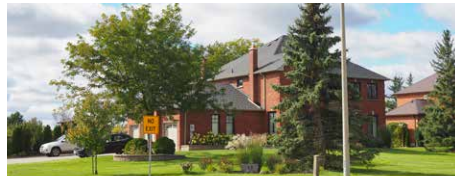
② Dwelling on Oak Ridge drive, adjacent to the subject site.
