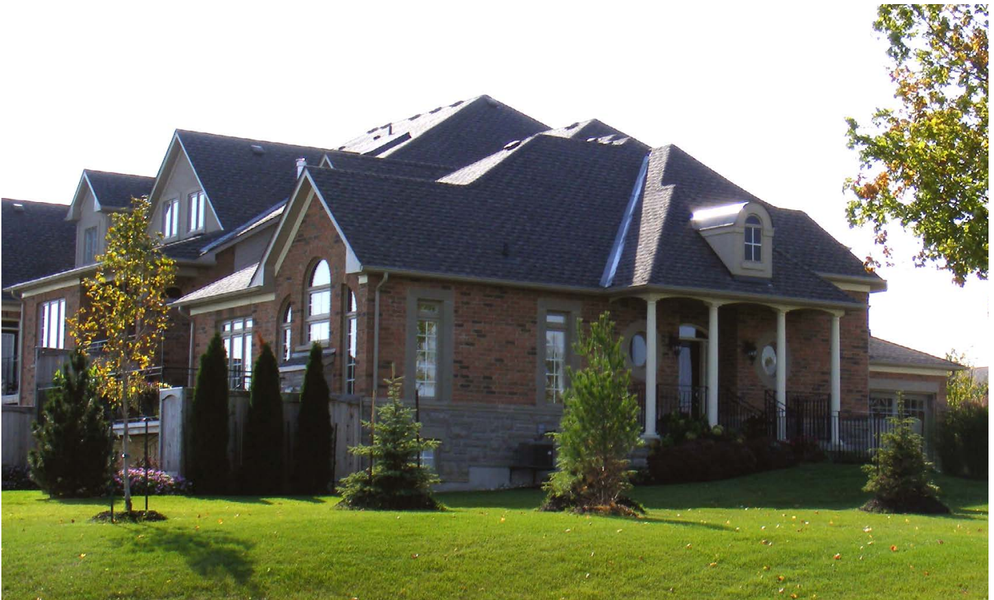
Figure 42 - Façades flanking/backing onto an open space should utilize a consistent level of architectural detail as front façades
