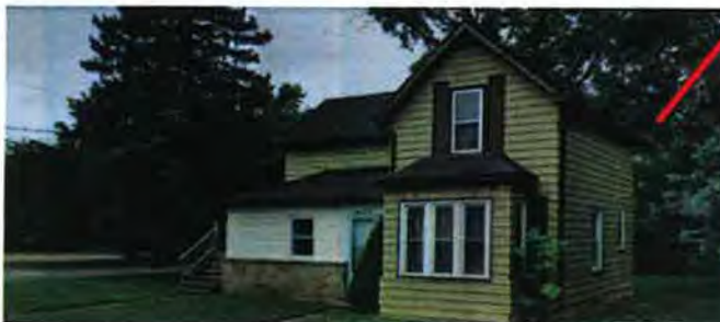
Figure 8 – WEST of Subject Property 22 Mill St. – Single Detached Home.
