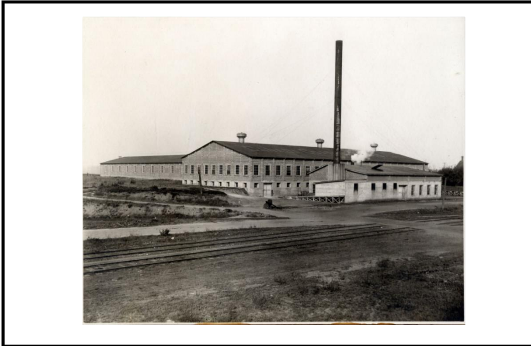
Figure 1: Canada Coated Paper Mill, ca. 1905 (EHS 1905)
