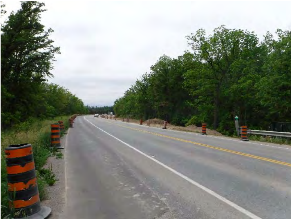
Photo 35. Trafalgar Road – View to west; current road widening works
