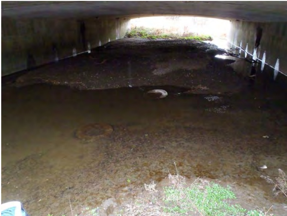
Photo 21. View under bridge facing downstream of main channel.
