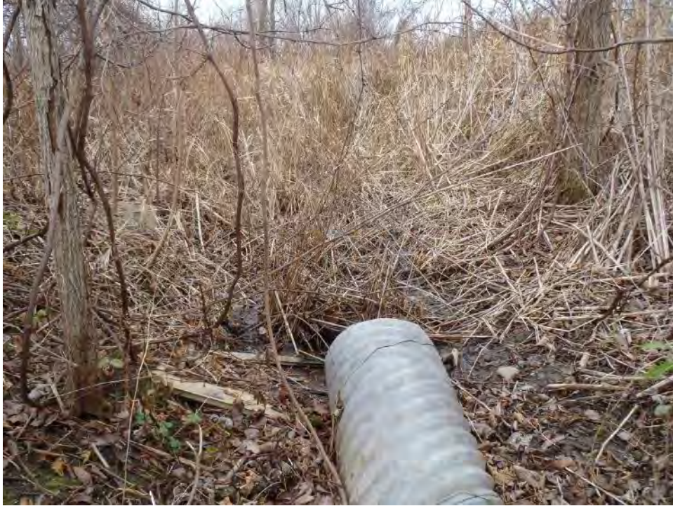
Photo 24. Downstream extent, looking upstream.
