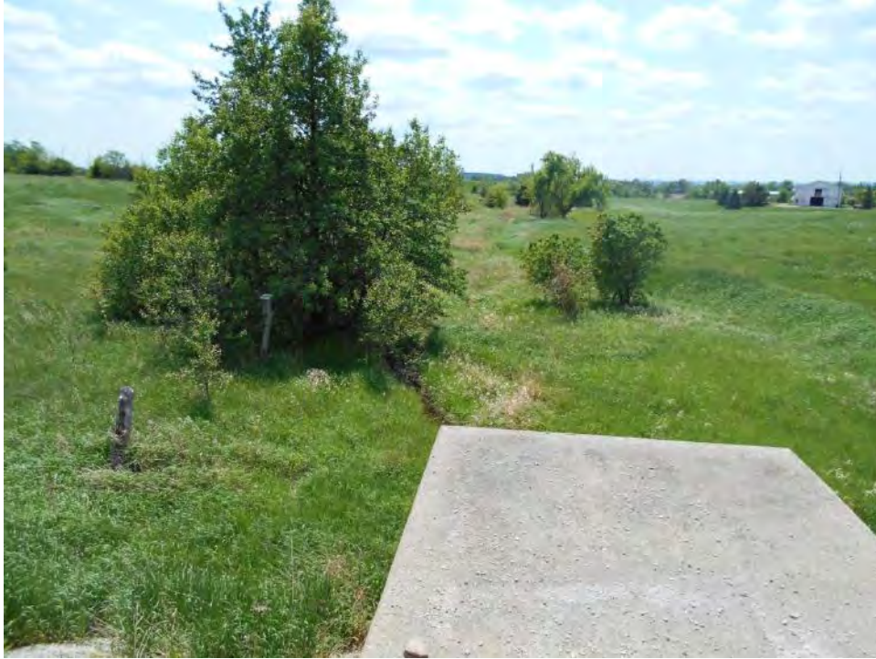
Photo 48. Looking downstream from road crossing.
